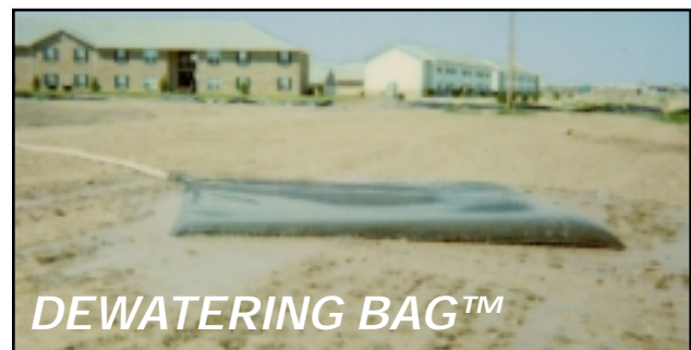
Sediment containment for pumped water
