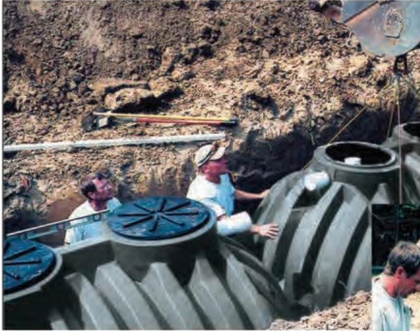
**5** Start addition of water and add approximately one foot more gravel mixture around the base of the tank. Continue to add the water at the same rate as the aggregate backfill material.
