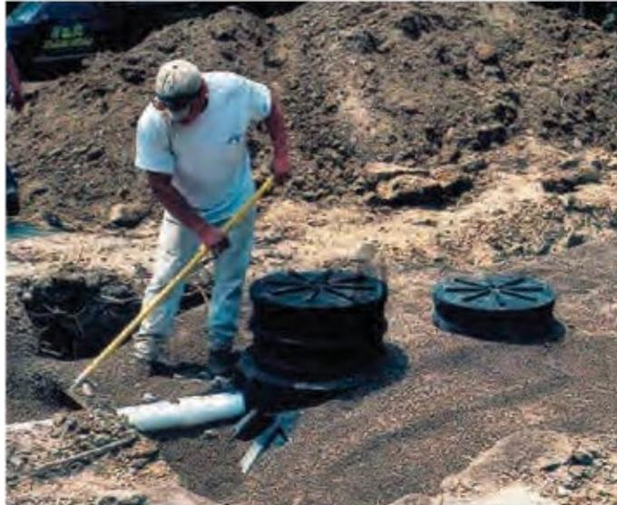
**7** Level-out the gravel and prepare for the final top soil. Approximately 6" deep. Install cover at this time.
