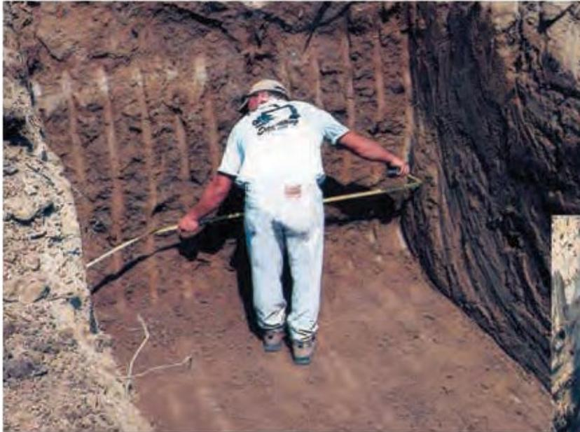
**1** Dig and measure for appropriate tank. Allow for an extra 6-12 inches of space around the tank. Maximum depth of bury is 24" from top of tank to finish grade.
