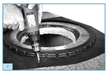
**8.** Install the EZsnap, EZset or TW-Risers and lids according to Infiltrator's Riser Guidance document.
