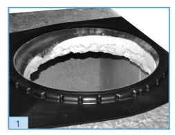
**1.** Position the Adapter Flange in place centered over manhole.
