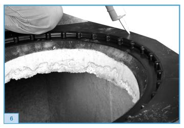
**7.** Fasten Adapter Flange to tank using (6) 1/4" x 1 1/4" (5.0 mm x 50 mm) stainless steel hex head tapcon screws with 1" x 3/8" stainless steel washers. Tighten in star pattern.
