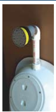
ODOR FILTER attaches to vent pipe to reduce sewer odors
