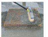
2. Remove sediment from the f of Inlet Filter.
