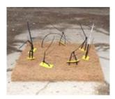
3. Position the mat. Place Inlet Filter on grate with the net side
