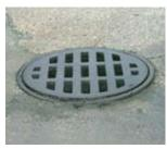
1. Remove sediment, debris, ice and snow from the inlet grate surface and surrounding area.
