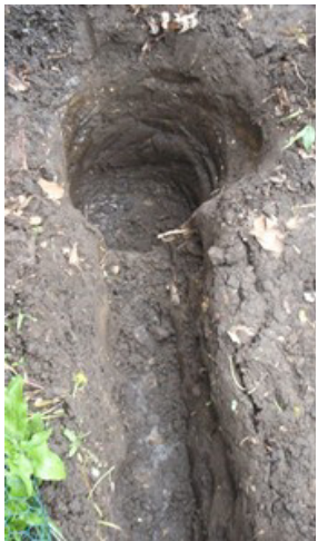
Excavate hole for drain sump and trench for drain pipe
